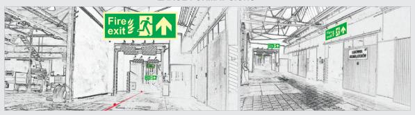
Large format signs are appropriate for use in large industrial facilities and production halls. Such solutions facilitate the evacuation. Our large format signs are produced on 5 mm PVC in normal version and are also available with photoluminescent overprints.
