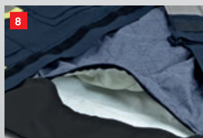
Inspection opening to check status of membranes
