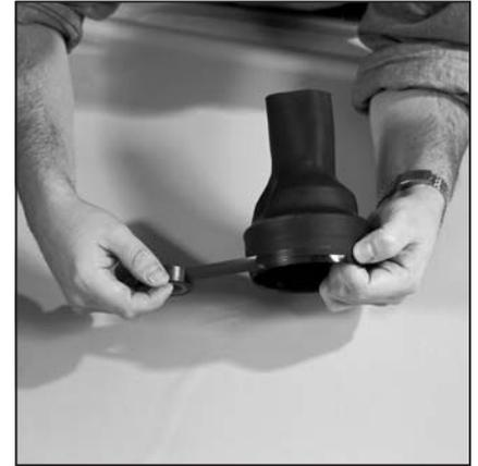
8. Fix the rubber cuff to the ring with tape going around the ring twice (two layers of tape).
