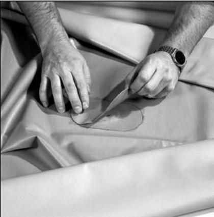
7. Apply the patch over the damage, starting from one end to avoid wrinkles.
