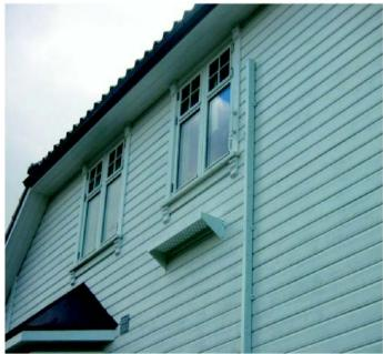
If the window opens "the wrong way" the escape ladder can be supplemented with an outdoor step.
