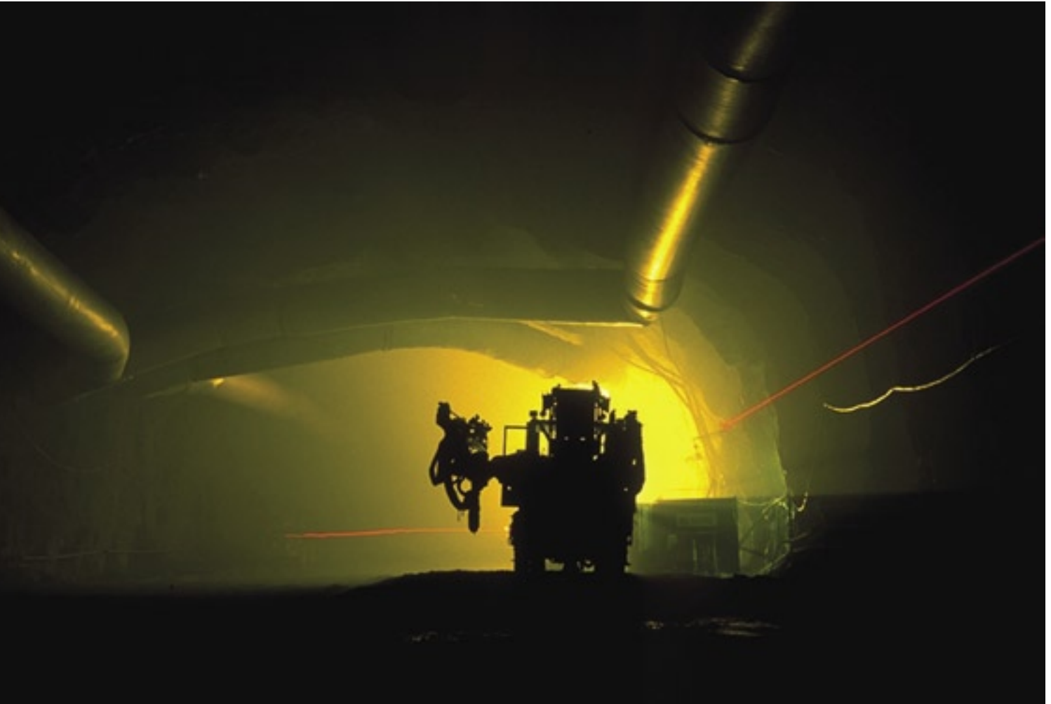
Tunnel under Arlanda
